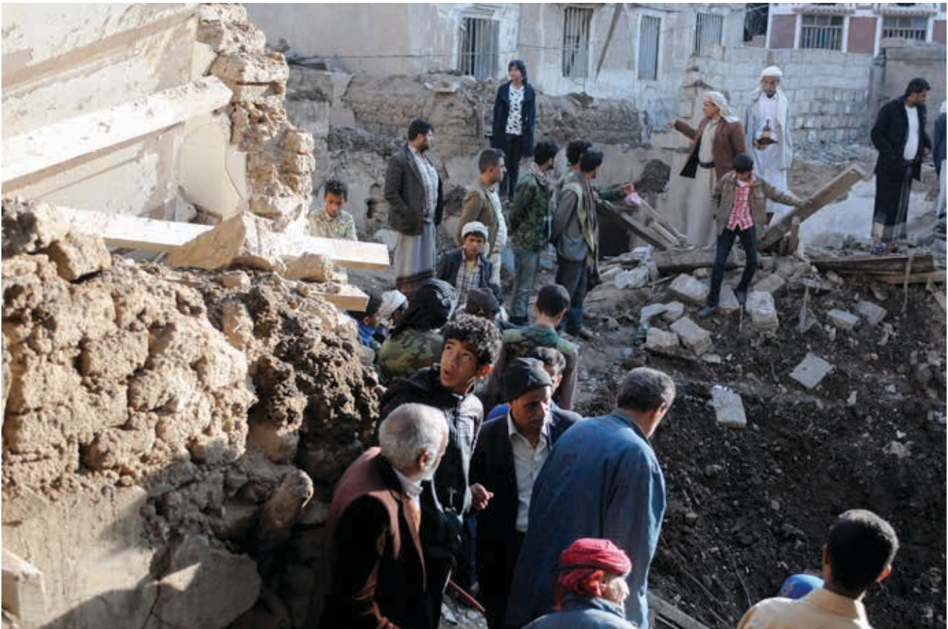
SANAA, YEMEN - NOVEMBER 11: People inspect wreckage of collapsed building after an air strike in the Yemeni capital of Sana'a on November 11, 2017. The Saudi-led military coalition carried out two air strikes on the defence ministry in Yemen's rebel-held capital Sanaa. © MOHAMMED HAMOUD / ANADOLU AGENCY
