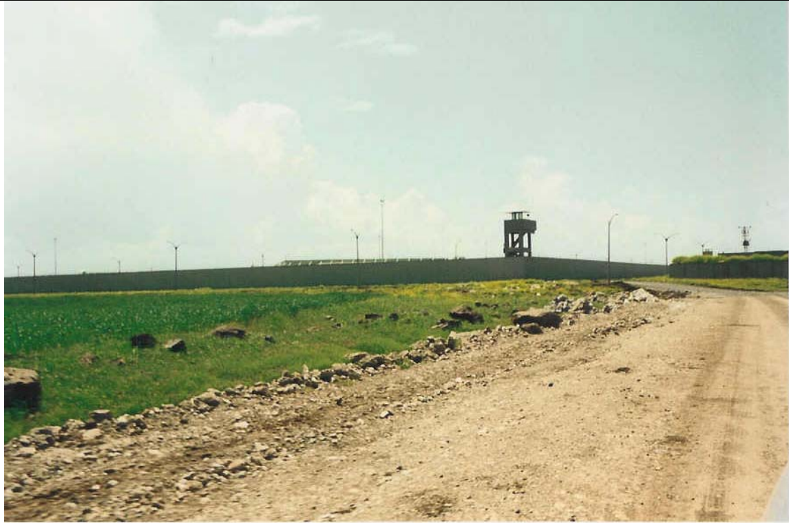
Photo: Newly-constructed High Security Prison, Diyarbakir province, Ücküyu village, Devegeçidi
