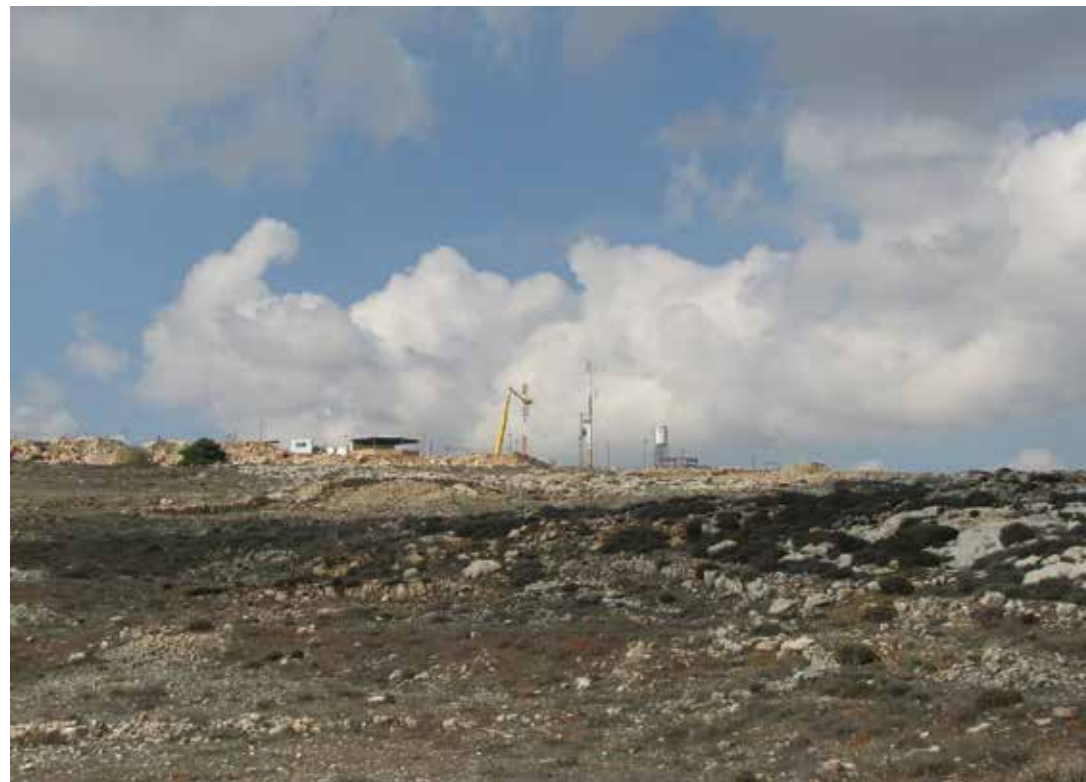
Partner Communications mast, located in the Migron outpost.
