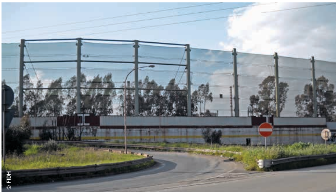
Protection installed to limit the diffusion of polluting dust
