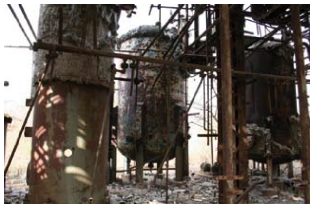
Bhopal: an environmental industrial catastrophe. A toxic cloud escaping from a chemical plant operated by a subsidiary of Union Carbide Company (USA) led to the death of more than 25 000 people. © CC-BY-SA-2.0. / Simone.lippi.
